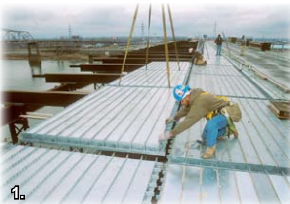
1. Setting the cast-in-place panels on the Eads River Bridge.
